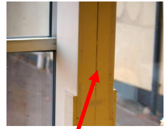
FIGURE 2: HAY LANE SCHOOL COLUMN. ARROW SHOWS ONE OF THE UNSEALED VERTICAL GAPS
